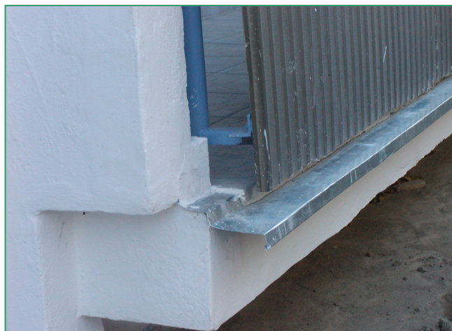
Detail lodžiovej dosky pri odkvape po obnove Detail of loggia board at the cornice following renovation
