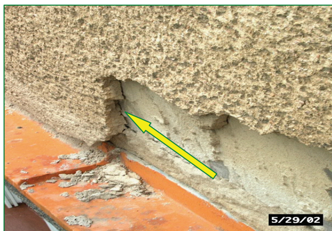
Odpadnutá a oddelená omietka hrúbky 40 mm pri rímse Fallen off and separated rendering with thickness of 40 mm at the moulding
